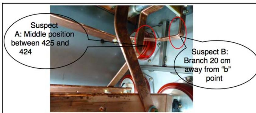
Figure 12. Suspected PD source location
